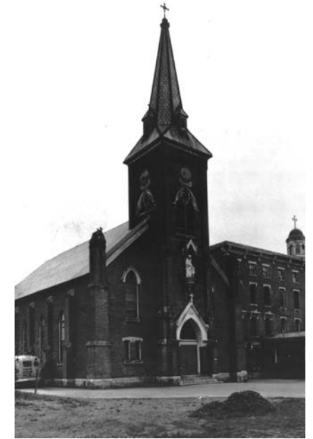
Historic St. Vincent's Church
